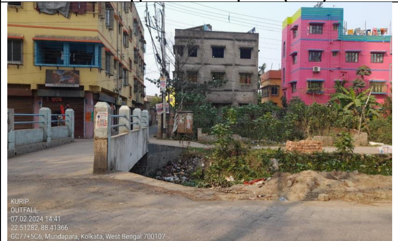
Outfall at Nazirbad(OF13)
