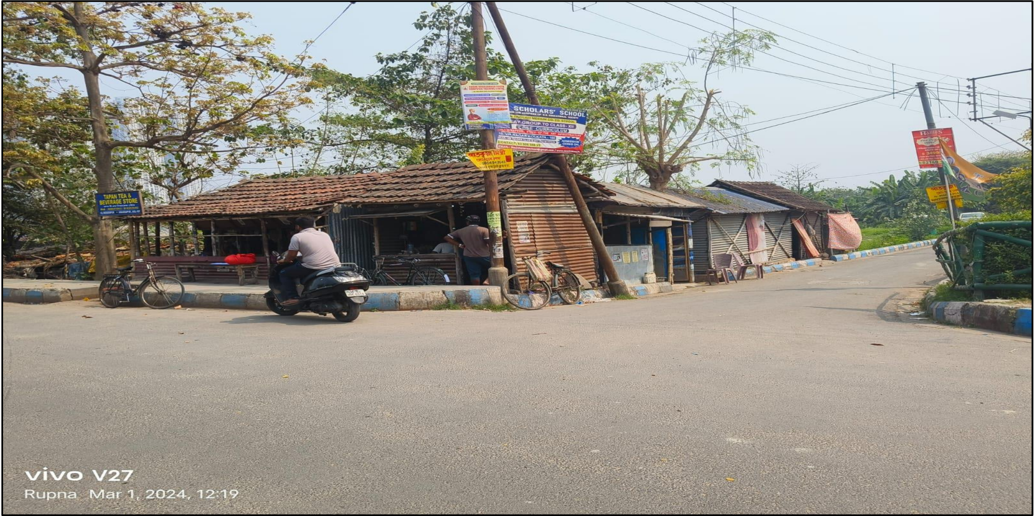
Photographs of Temporarily affected shops at the entry point of the Proposed Pumping Station
