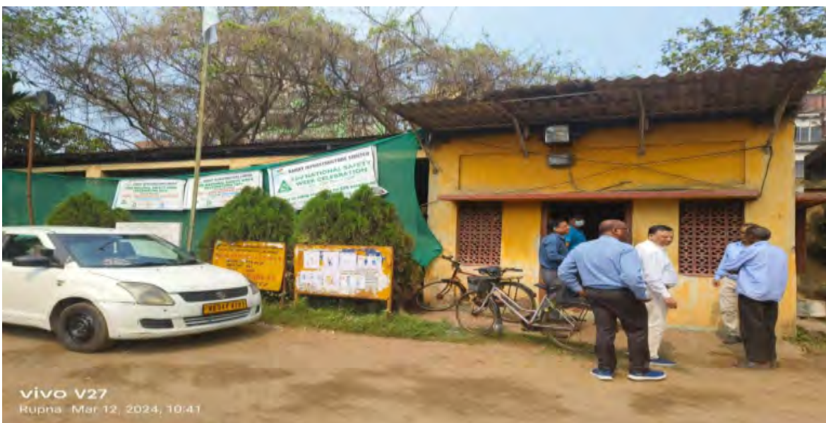
Photograph of PWD Section Office
