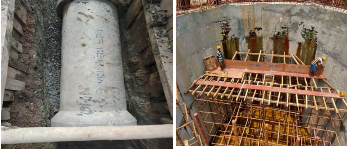
Project Location and Activity initiated by Contractors in SD-31LOT1 and SD-34
