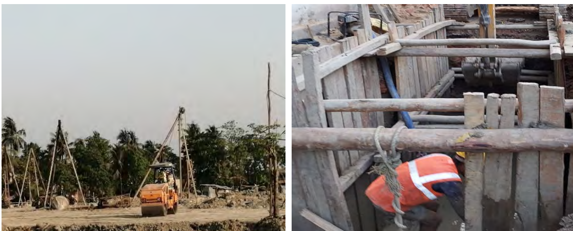
Project Location and Activity initiated by Contractors in SD-29 and SD-27R
