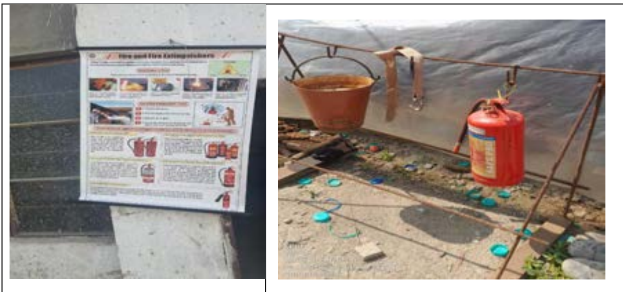
Fire Extinguishing Training Posters and fixed fire extinguisher near the DG room and main panel room
