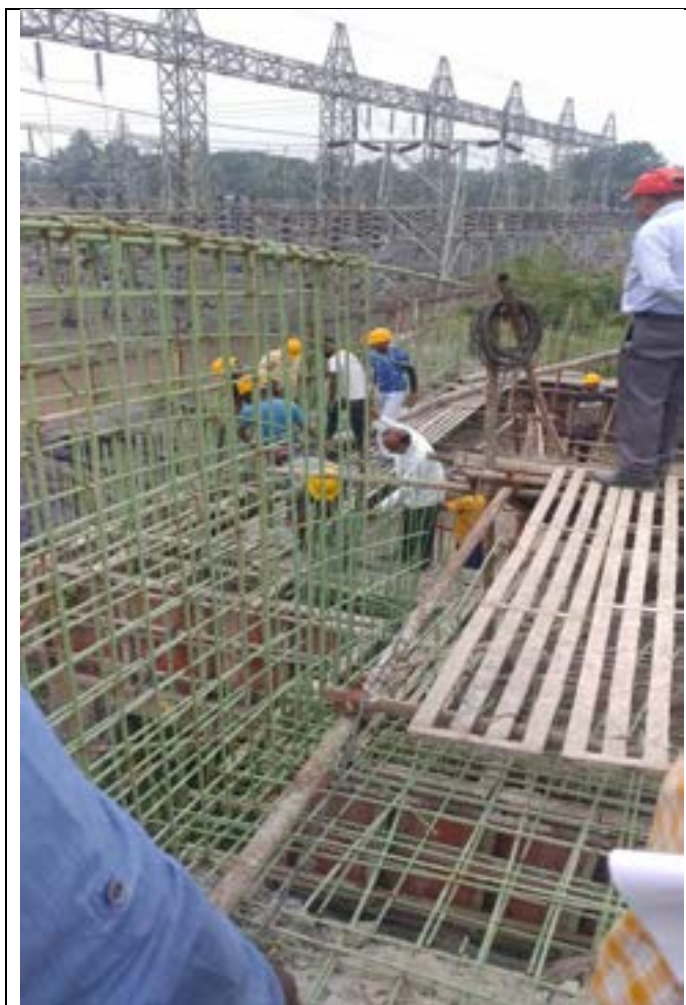
Figure 9: Laundry base slab shuttering & reinforcement work are under progress in SD28
