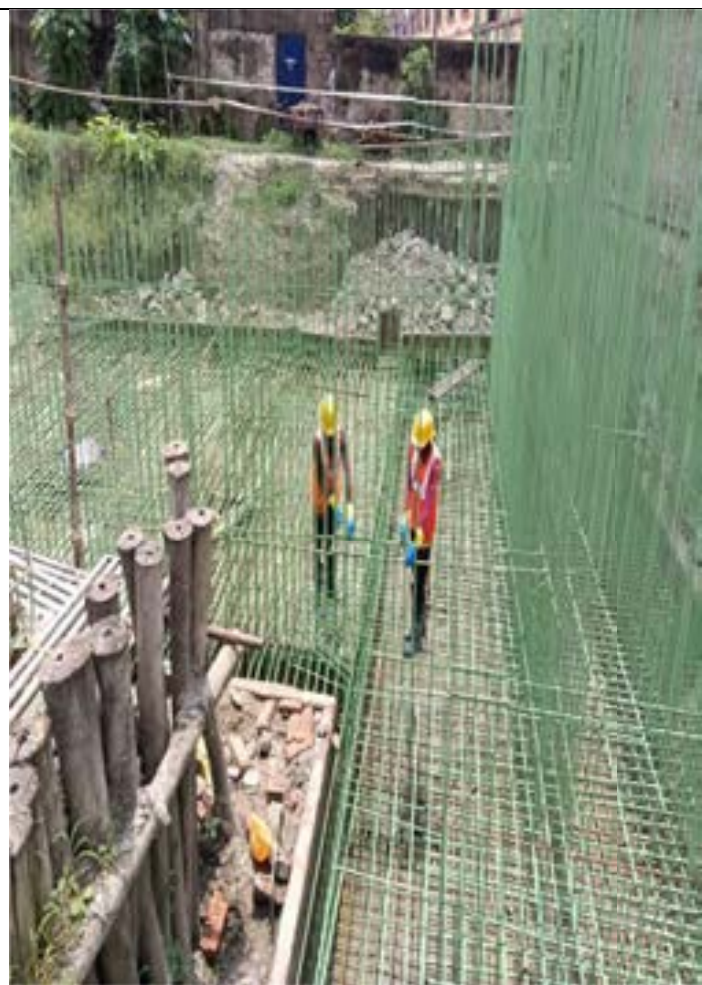
Figure 10: Laundry base slab shuttering & reinforcement work are under progress in SD29
