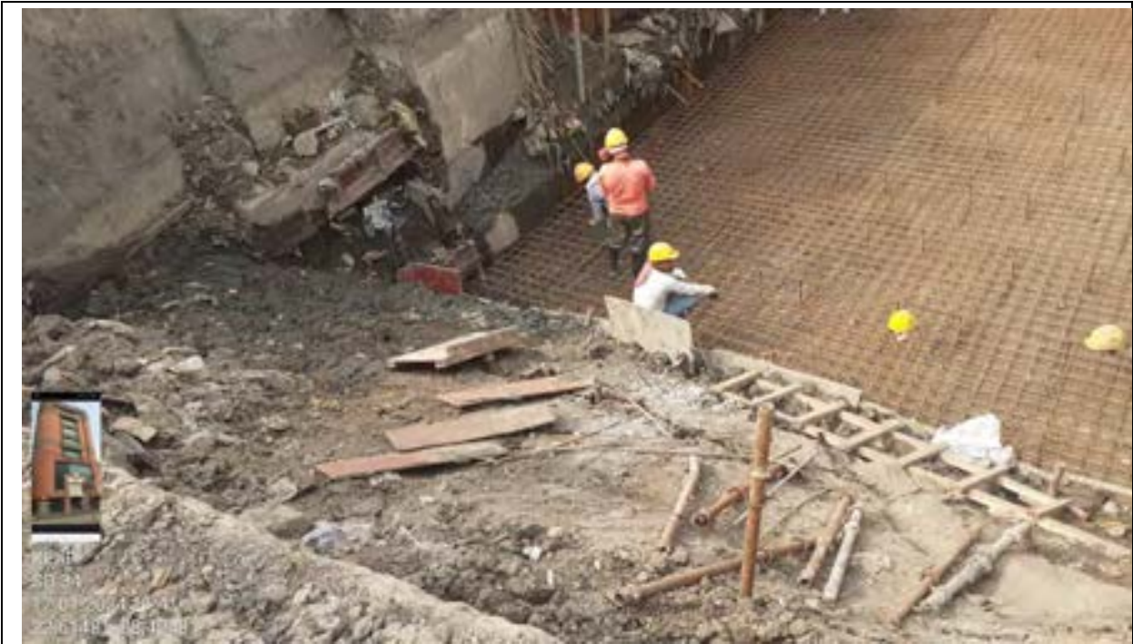
Figure 15: RCC concrete work is in progress at Lalababu site in SD 34
