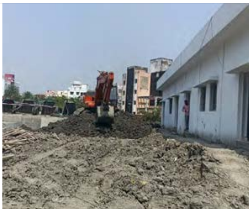
Figure 14: Excavation work is in progress at Mukundapur in SD 32
