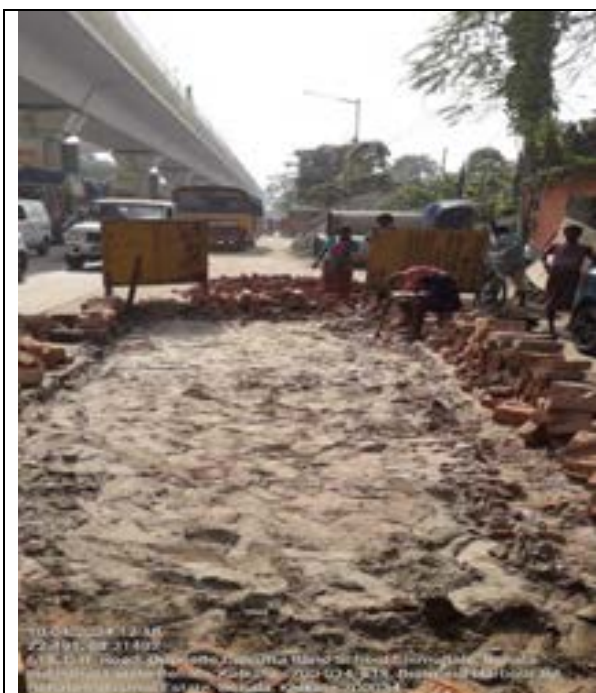
Figure 13: Road restoration work in progress at D.H. road in SD 31R2
