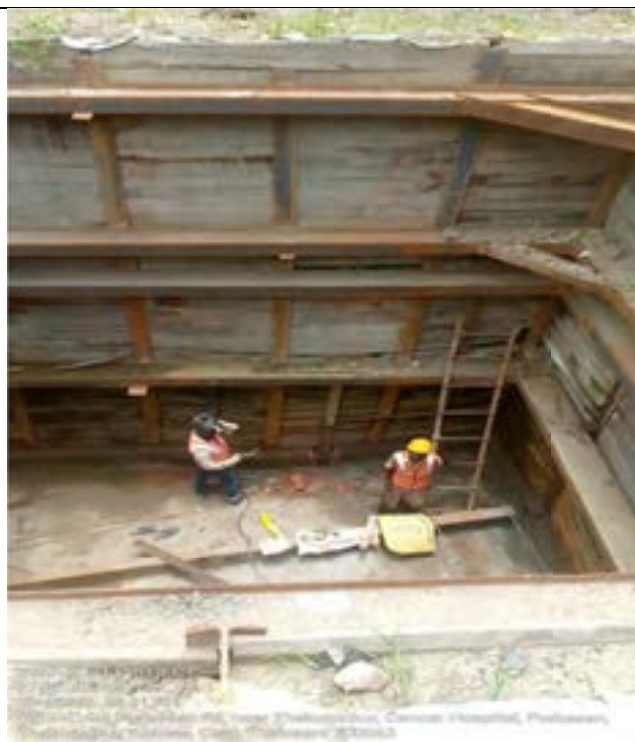
Figure 12: Welding activities in progress in SD 31LOT1
