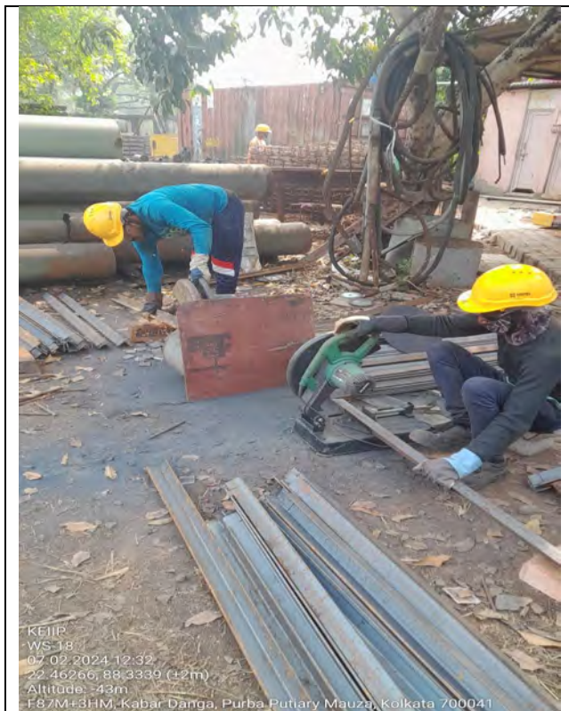
Construction work in progress at Kabar Danga (WS-18)
