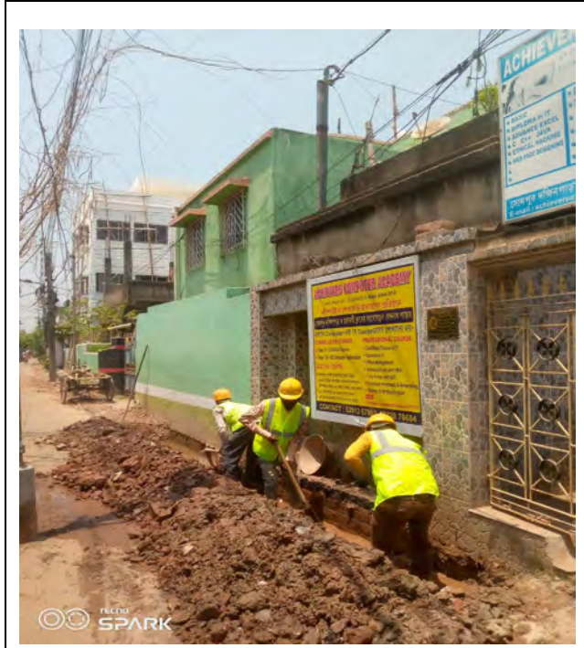
MS Pipe Welding works at Prantik MG Road (WS- 17A)
