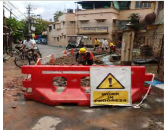
Barricading of the excavated area
