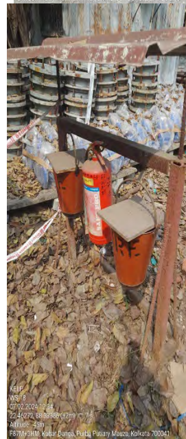
Fire safety at site
