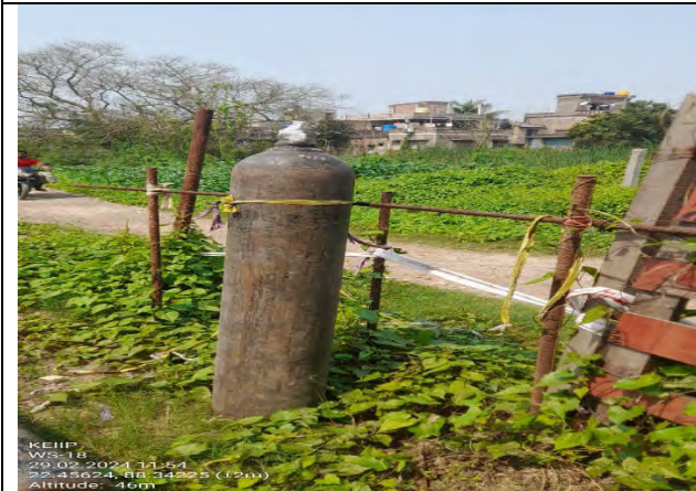
Secure cylinders in an upright position
