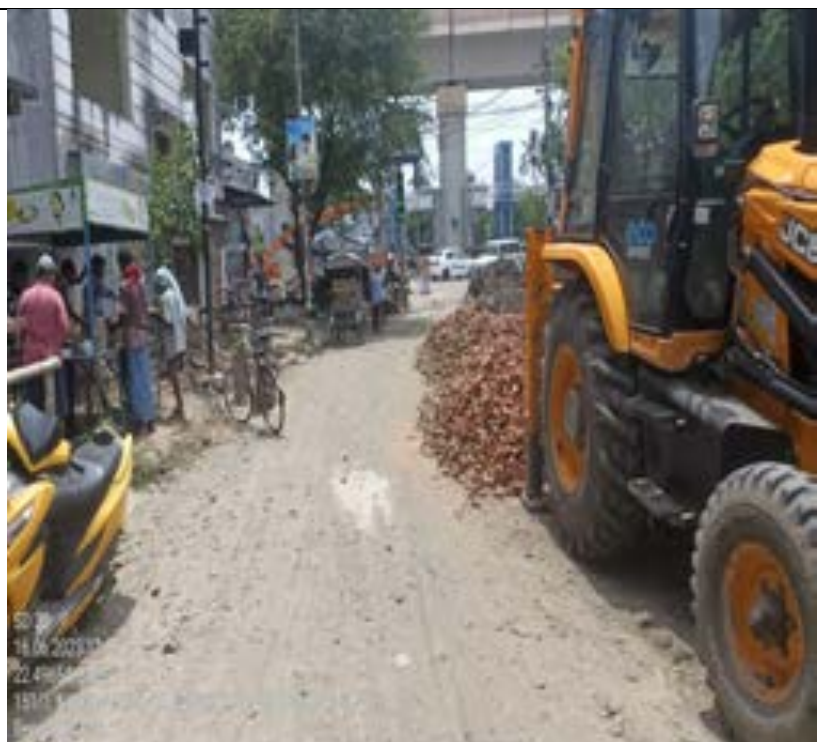
Figure 14: Road restoration work is in progress at Mukundapur in SD 32
