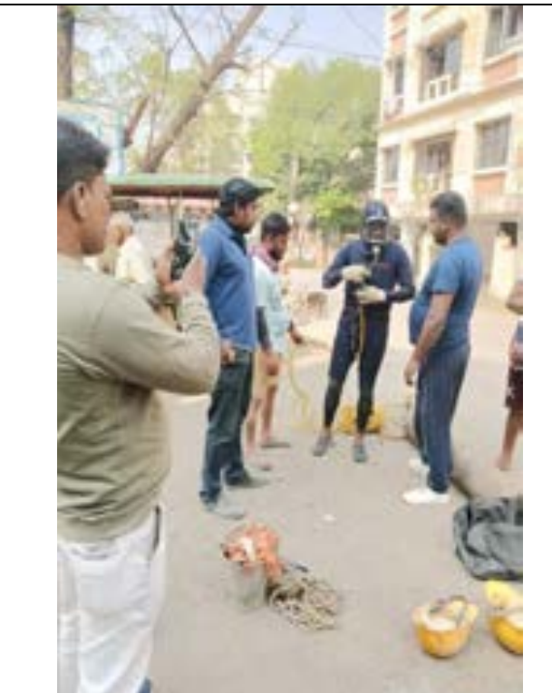
Use of safety arrangement with proper PPEs for manhole seal breaking
