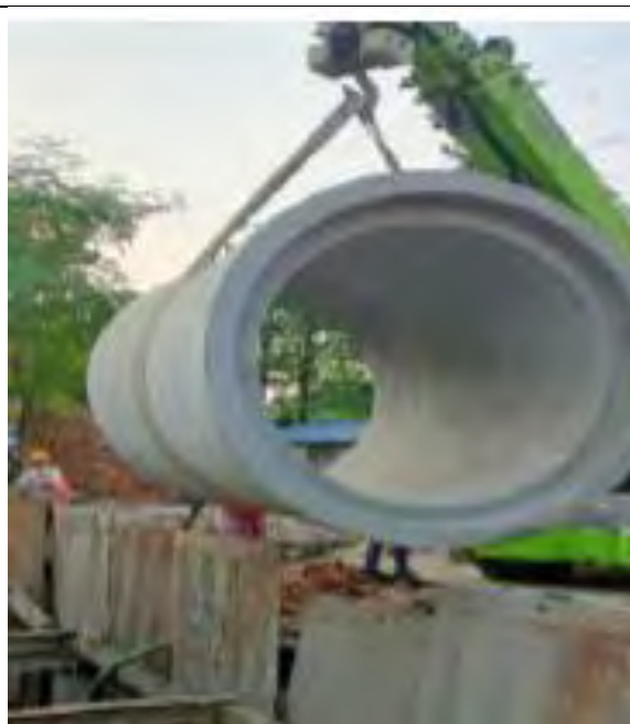
Figure 12: Safe pipe laying activities in progress in SD 31LOT1
