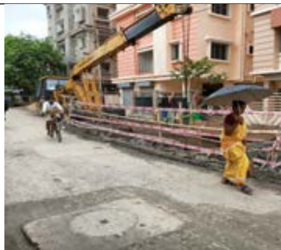
Barricading approach for public safety
