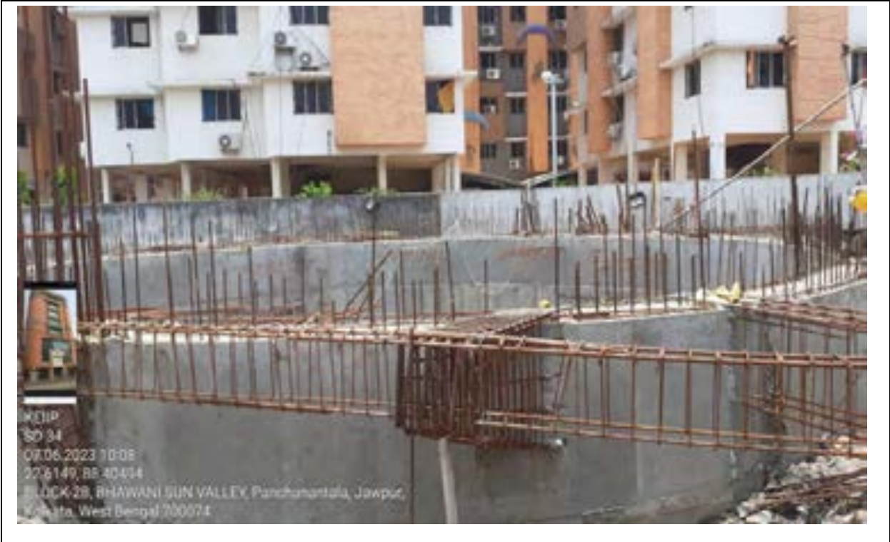
Figure 15: PH column reinforcement at Lalababu site in SD 34
