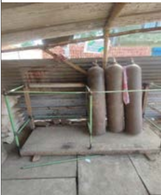
Secure cylinders in an upright position
