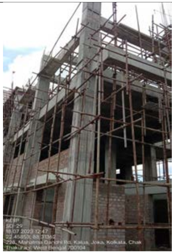
Figure 10: Casting of columns of main building in SD29
