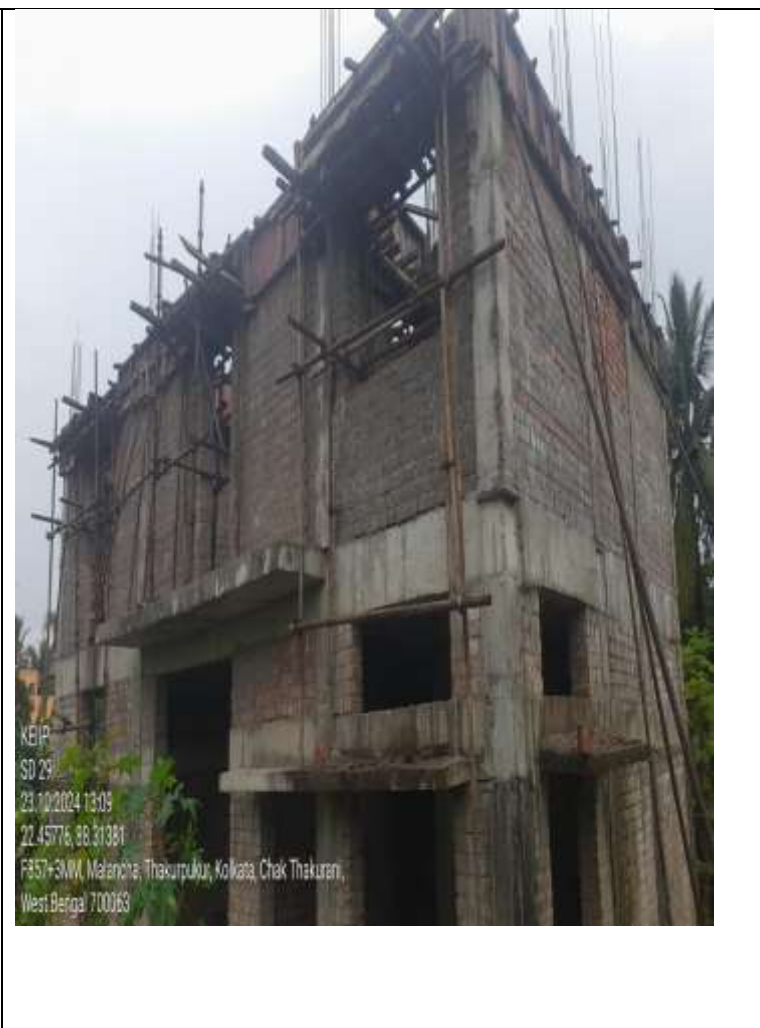
Figure 10: Launder base slab shuttering & reinforcement work are under progress in SD29
