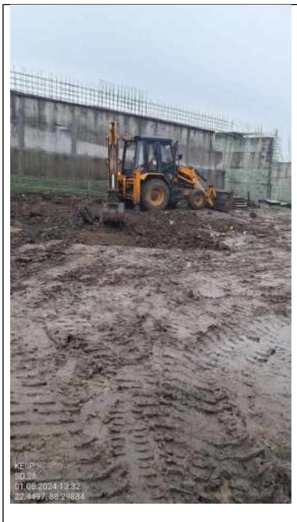
Figure 9: Excavation work is in progress at Joka in SD28
