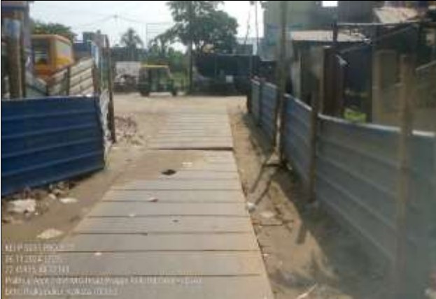
Steel sheet road surface with hard barricading at project site
