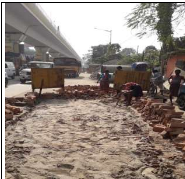
Figure 13: Road restoration work in progress at D.H. road in SD 31R2
