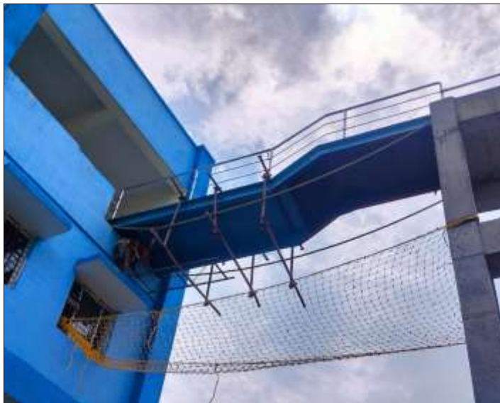
Figure 11: safety net during construction of admin building in SD30R
